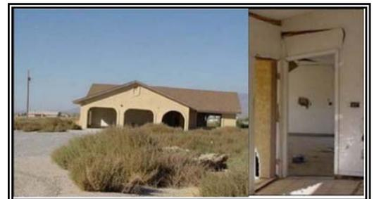
*A House in Nevada Damaged by Land Subsidence and an Earth Fissure*
